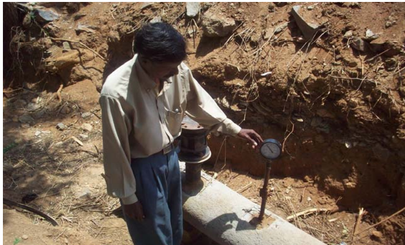
Third Party agency witnessing pressure test of pipelines
