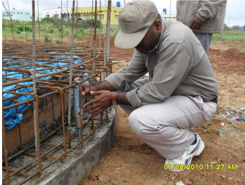
Third Party agency performing tests at site
